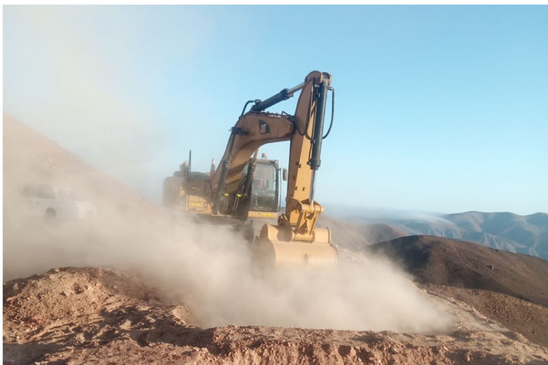
Picture 1. Road building in the new Lourdes-Condori drilling areas of the Los Chapitos copper project.
